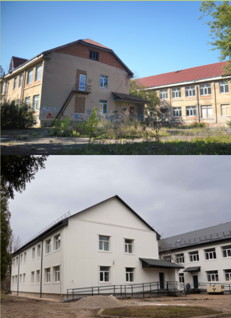
The facades of the former kindergarten "Zirochka" in Kalush before and after renovation
